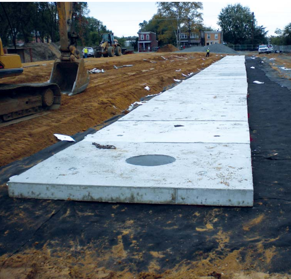
Completed stormwater system installed with manhole for chamber access.
