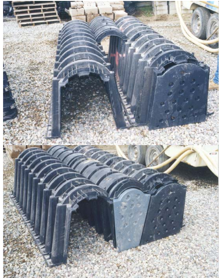
Figure 1. Storm water detention system components as assembled.
